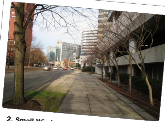
2. Small Windows, Screened Garages, or Blank Walls with Design Attributes – Some buildings have limited opportunities to see into their interior or for signage that gives passerbys a sense of what is going on inside. Screened parking mitigates some of the negative impacts of parking but certainly does not enhance the streetscape.
