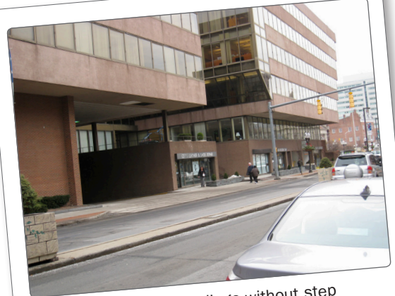
Even when short, buildings without step backs and particularly those with overhangs overwhelm the sidewalk and detract from the pedestrian experience
