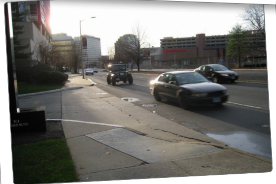
In addition to interruptions, drop-down ramps often lead pedestrians, strollers, and wheelchairs into the path of traffic (Tresser Boulevard)
