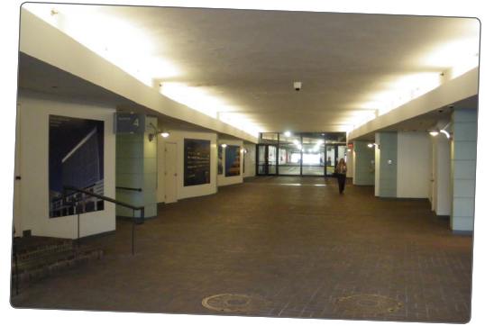
Though wide, a lack of natural light or informational signage reduce the utility and attractiveness of the passageway
