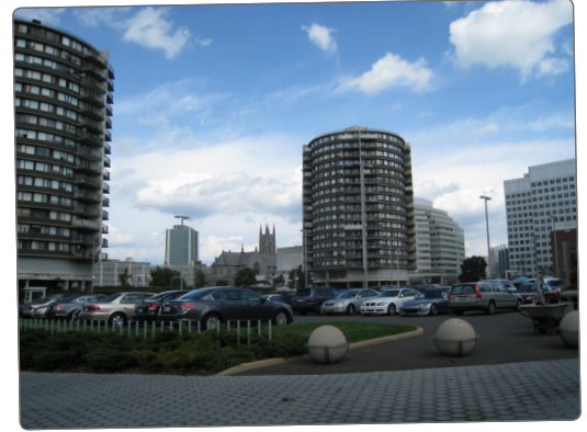
UBS phase IV site from Washington Boulevard, shown sandwiched between office and residential uses (B)
