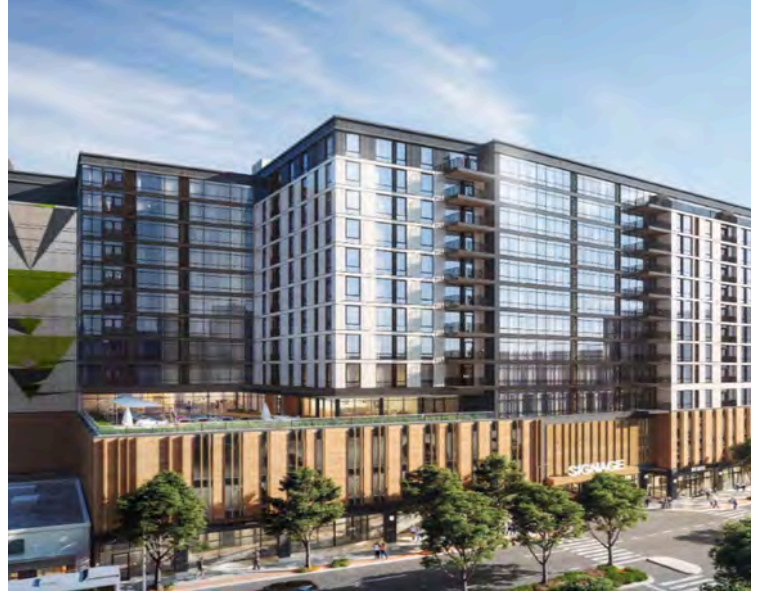
THE COASTLINE 130 Broad Street 200 residential units TR Broad II LLC
