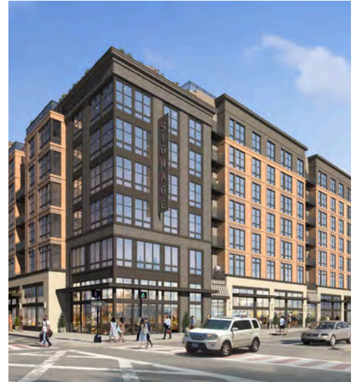
74 Broad 74 Broad Street 280 residential units and 5,400 sq ft of retail RMS 74 Broad Street, LLC
