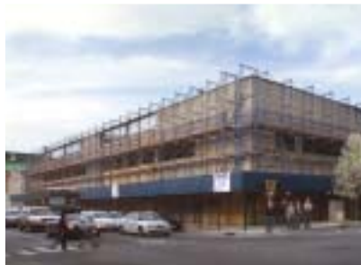
Burlington Coat Factory (in construction)
